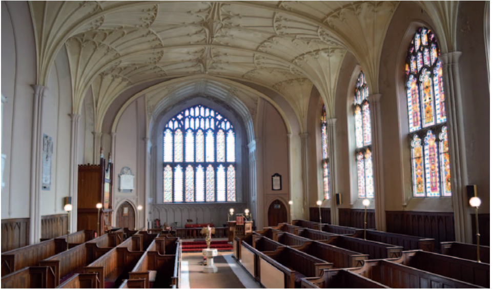
Fan vaulting at Collon Church
