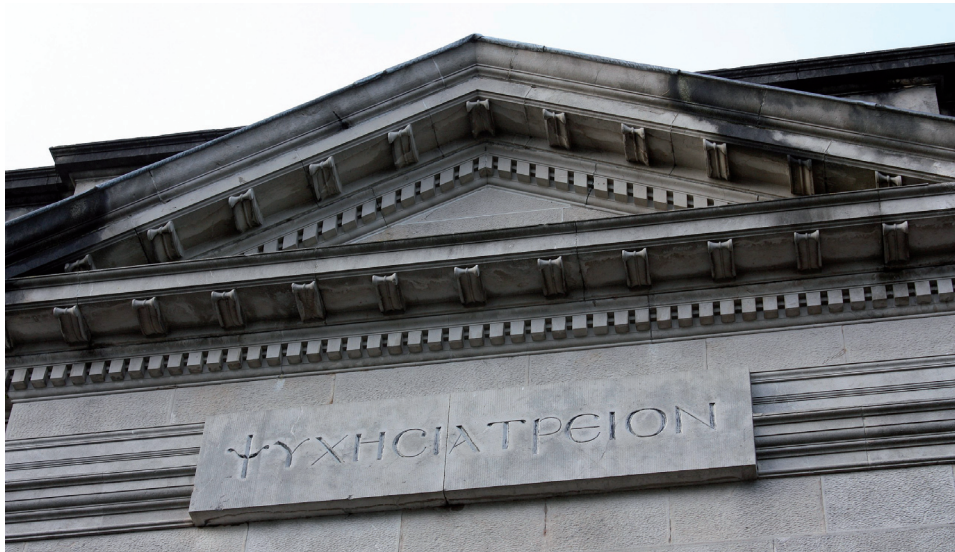
The Greek inscription on the façade of the Library building
